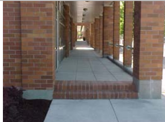
South Side Pedestrian walkway looking east.
