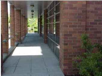
South Side Pedestrian walkway looking west.
